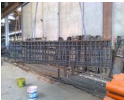
Figure 8 Positioning the template in the reinforcement cage of the plinth before casting the foundations
