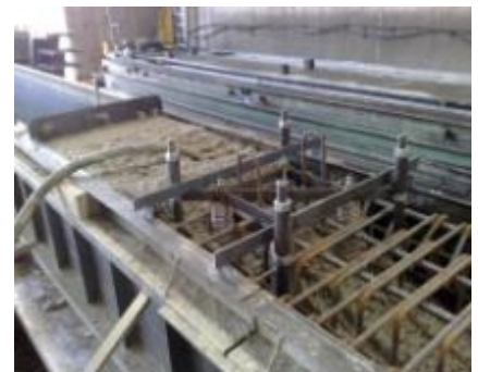
Figure 8 Positioning the template in the reinforcement cage of the plinth before casting the foundations
