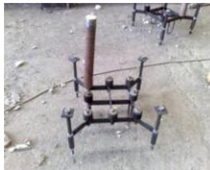
Figure 8 Positioning the template in the reinforcement cage of the plinth before casting the foundations
